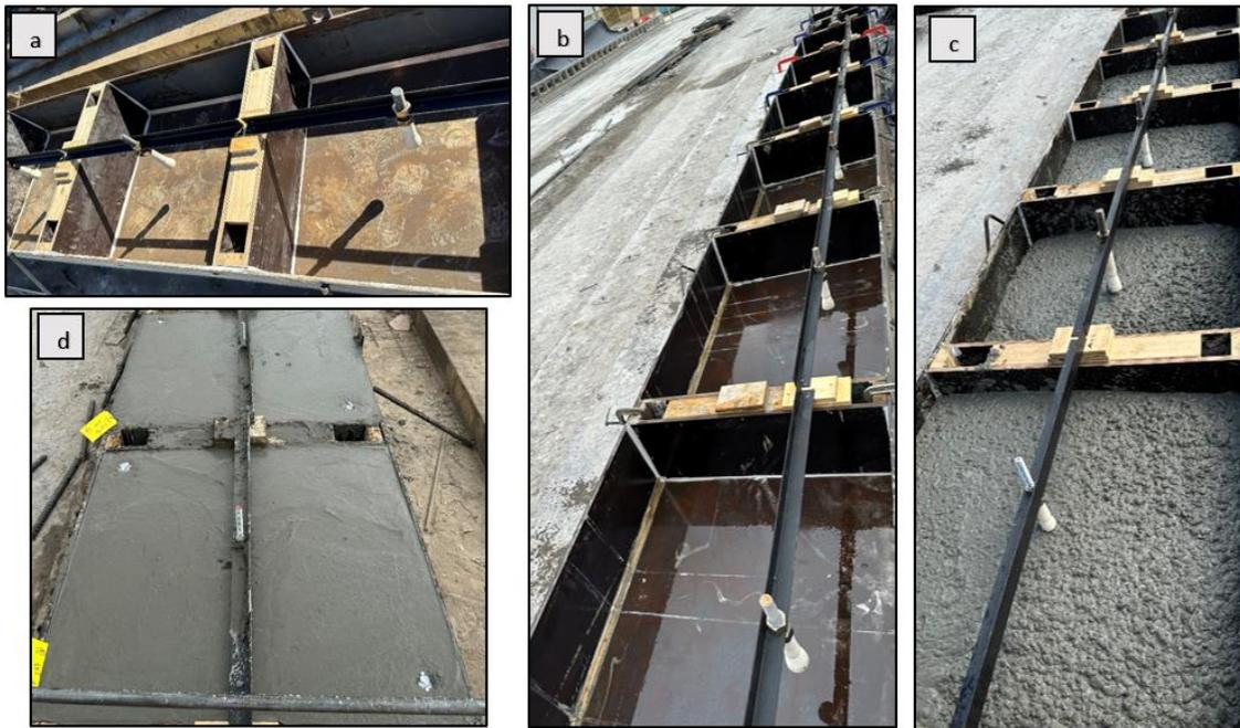
**Figure 11.** a) Adjustment of the specimen forms and position of the insert; b) casting bed cleaned and sprayed with lubricant; c) concrete being poured into the forms; d) position of the lift inserts.
