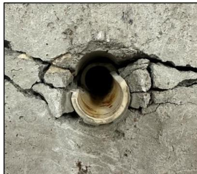
**Figure 29.** FCI insert fracture at the top.
